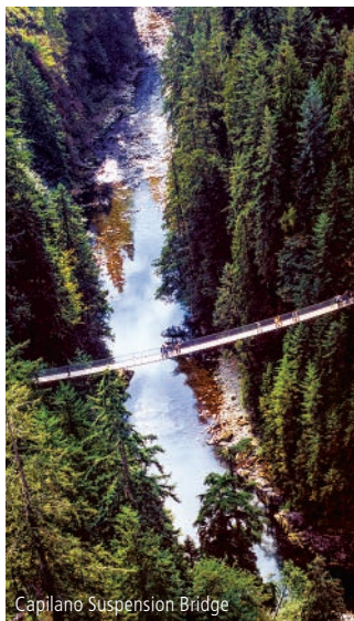
Capilano Suspension Bridge
